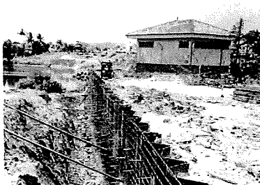
Sheet pile wall construction
