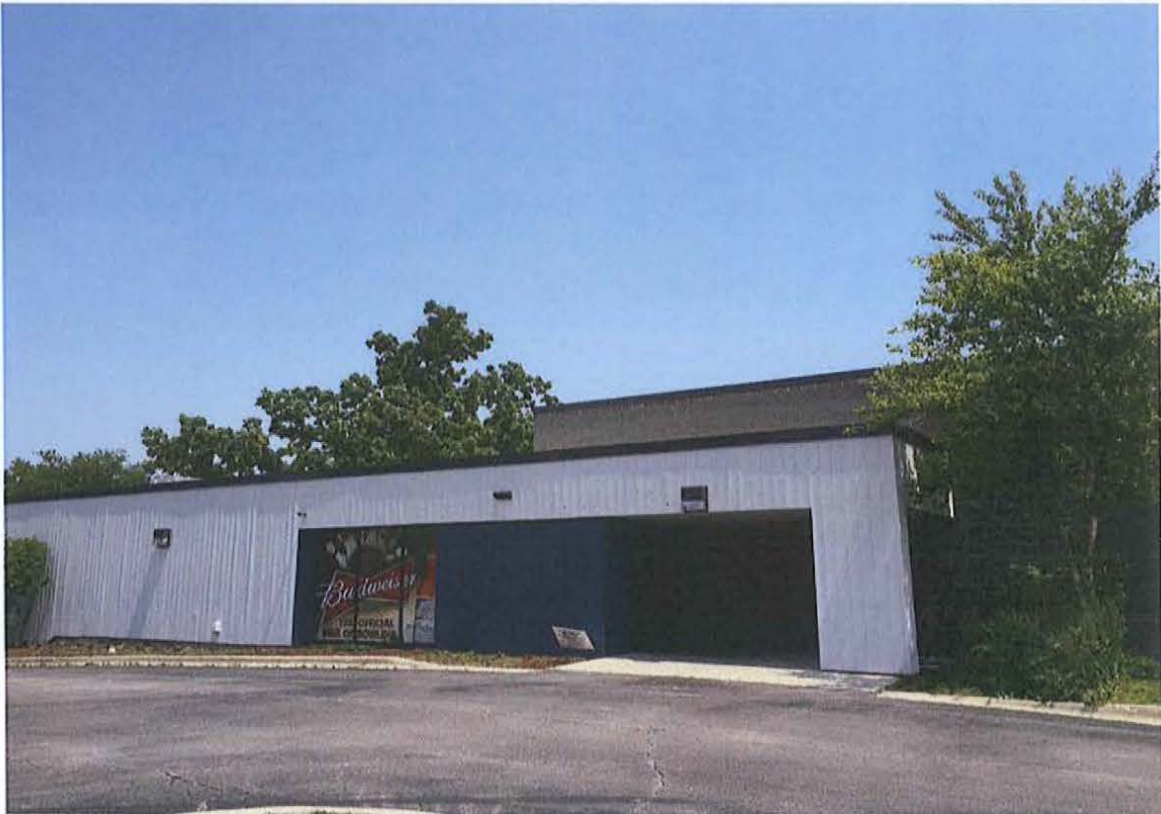
Main Bowling Center Entrance / Parking Lot Side (West)
