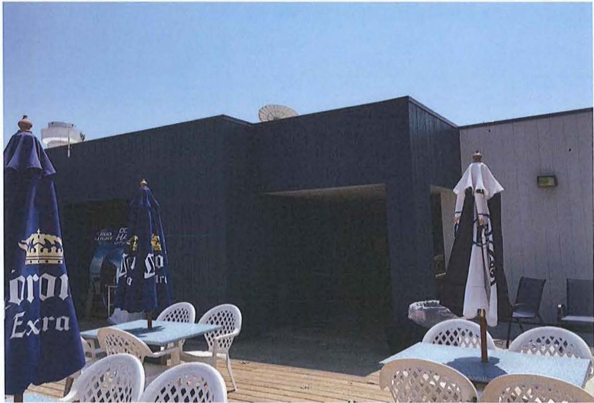
Finished Paint / Back of Building (North)
