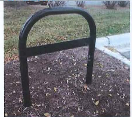
'U' Racks are 34" High 1.90" and 2 3/8" OD Steel Tubing and 3/8" Flat Bar
