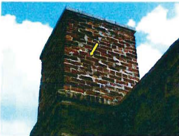
FR.61 / North Elevation, Deteriorated Chimney Masonry, All Elevations.
