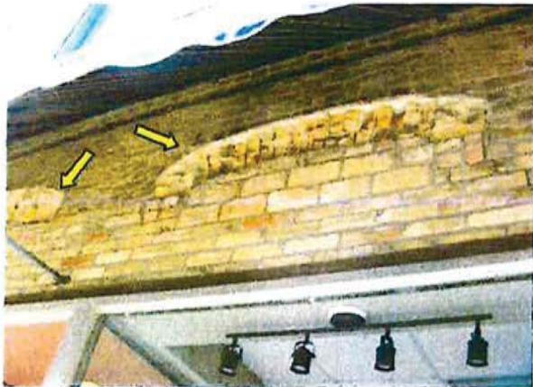
FR.21 / Main (East) Street Elevation, Level One Removed Masonry Arch.
