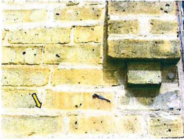
FR.52 / South Elevation, Masonry Pointing Required, Floor 2.
