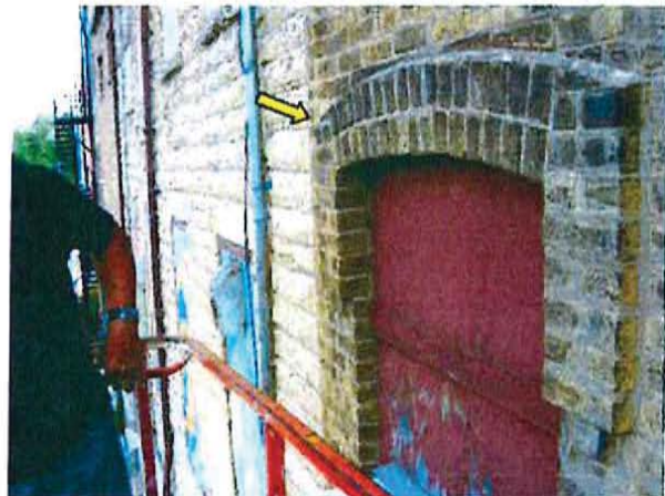
FR.40 / Turner (West) Court Elevation, Masonry Pointing, Required, Floor 1 (North) Above Grade Level.
