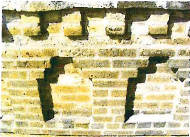
FR.11 / Main (East) Street Elevation, Masonry Corbel-Table with Masonry Dentils in the Bed Mould of the Cornice.
