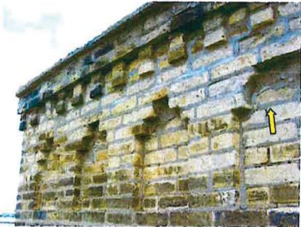
FR.29 / Turner (West) Court Eleva., Masonry Corbel-Table with Masonry Dentils in the Bed Mould of the Cornice.
