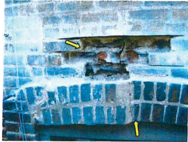
FR.33 / Turner (West) Court Elevation, South Inspection Opening, Floor 2. Masonry Arch Distress.
