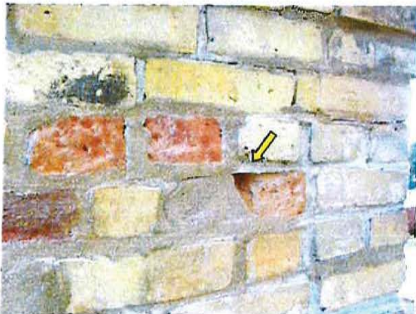
FR.34 / Turner (West) Court Elevation, Deteriorated Repair, South Corner, Floor 3 @ Head.
