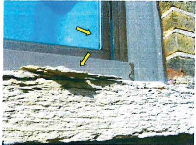
FR.13 / Main (East) Street Existing Deteriorated Sandstone Window Sill. Replacement Aluminum Windows.
