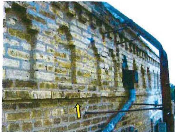
FR.30 / Turner (West) Court Eleva., Masonry Corbel-Table with Masonry Dentils in the Bed Mould of the Cornice.
