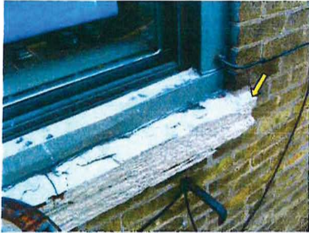
FR.37 / Turner (West) Court Elevation, Existing Deteriorated Sandstone Window Sill, North, Floor 3.
