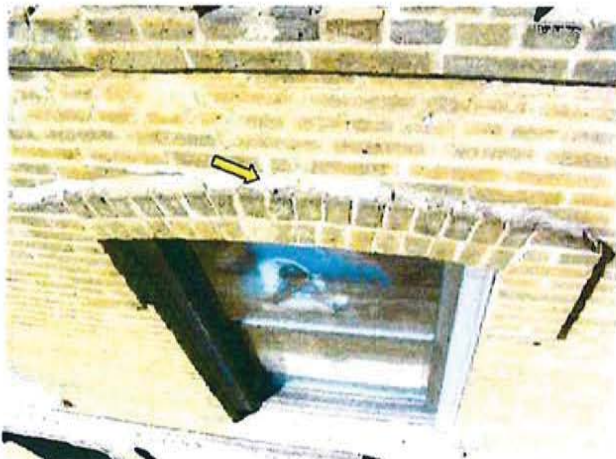
FR.14 / Main (East) Street Elevation, Curved Masonry Segmental Window Arch, Two Rowlock Header Courses.
