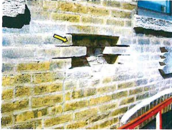
FR.22 / Main (East) Street Elevation, South Inspection Opening, Floor 3.
