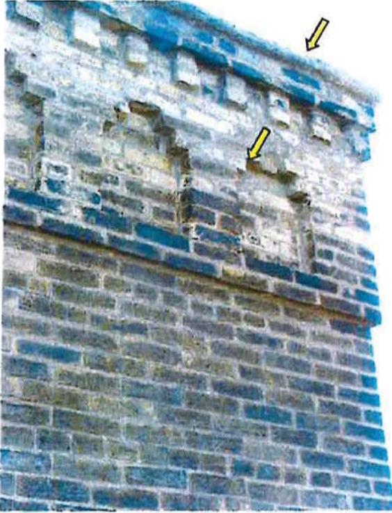
FR.62 / North Elevation, Deteriorated Limestone Cap & Masonry.
