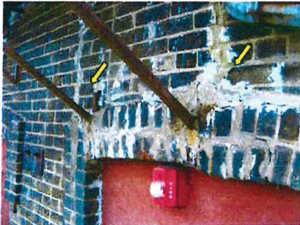
FR.39 / Turner (West) Court Elevation, Deteriorated Repair, Floor 1 Above Grade Level @ Fire Escape.
