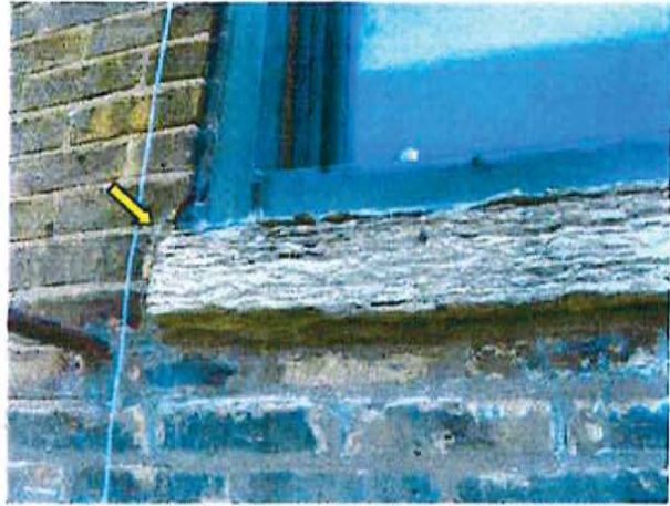
FR.38 / Turner (West) Court Elevation, Existing Deteriorated Sandstone Window Sill, South, Floor 3.
