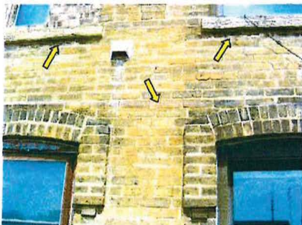
FR.41 / South Elevation, Deteriorated Limestone Sills, Masonry Pointing Required.
