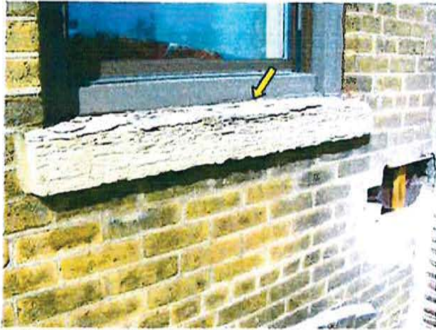
FR.12 / Main (East) Street Existing Deteriorated Sandstone Window Sill.
