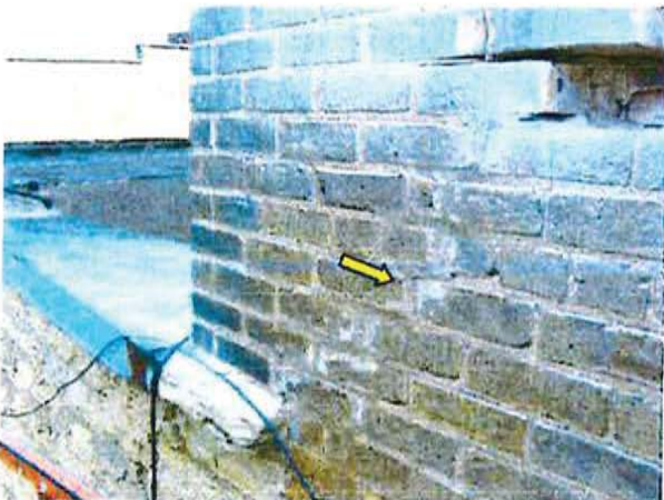
FR.31 / Turner (West) Court Elevation, Masonry Stress, Floor 3 (North),
