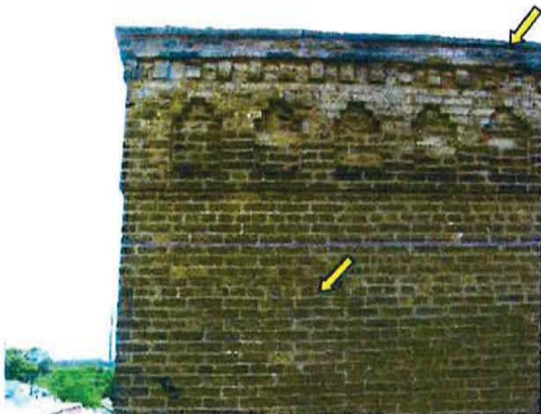
FR.56 / North Elevation, Masonry Pointing Required, Floor 3. Deteriorated Limestone Sill.
