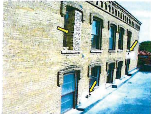
FR.43 / South Elevation, Masonry Infill @ Removed Window. Inspection Openings, Floor 2 & 3.
