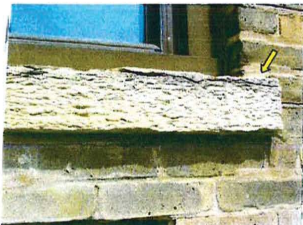
FR.51 / South Elevation, Deteriorated Limestone Sill, Floor 3.
