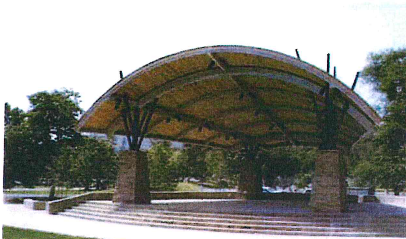
Bandshell Character - Barrel Roof, Custom Metal Supports, Limestone Wrapped Columns
