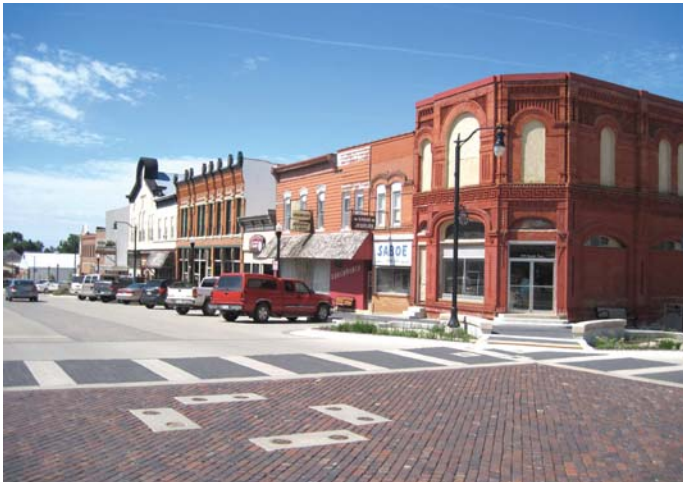
Original brick pavers from 1914 were recovered and re-used in the intersections
