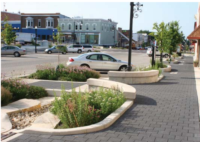
Porous paving and rain garden planters beautify the sidewalks
