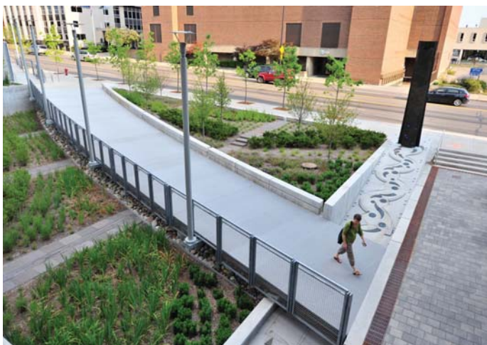
The path of rain water is displayed artfully using decorative runnels
