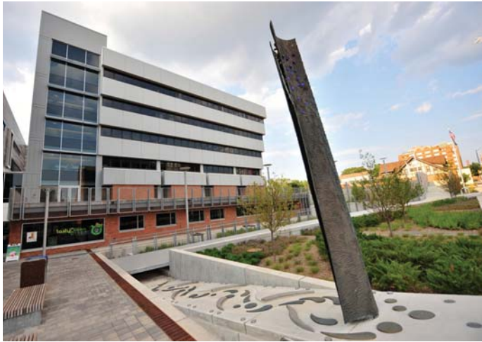
Rainwater art in plaza of Ann Arbor Municipal Center
