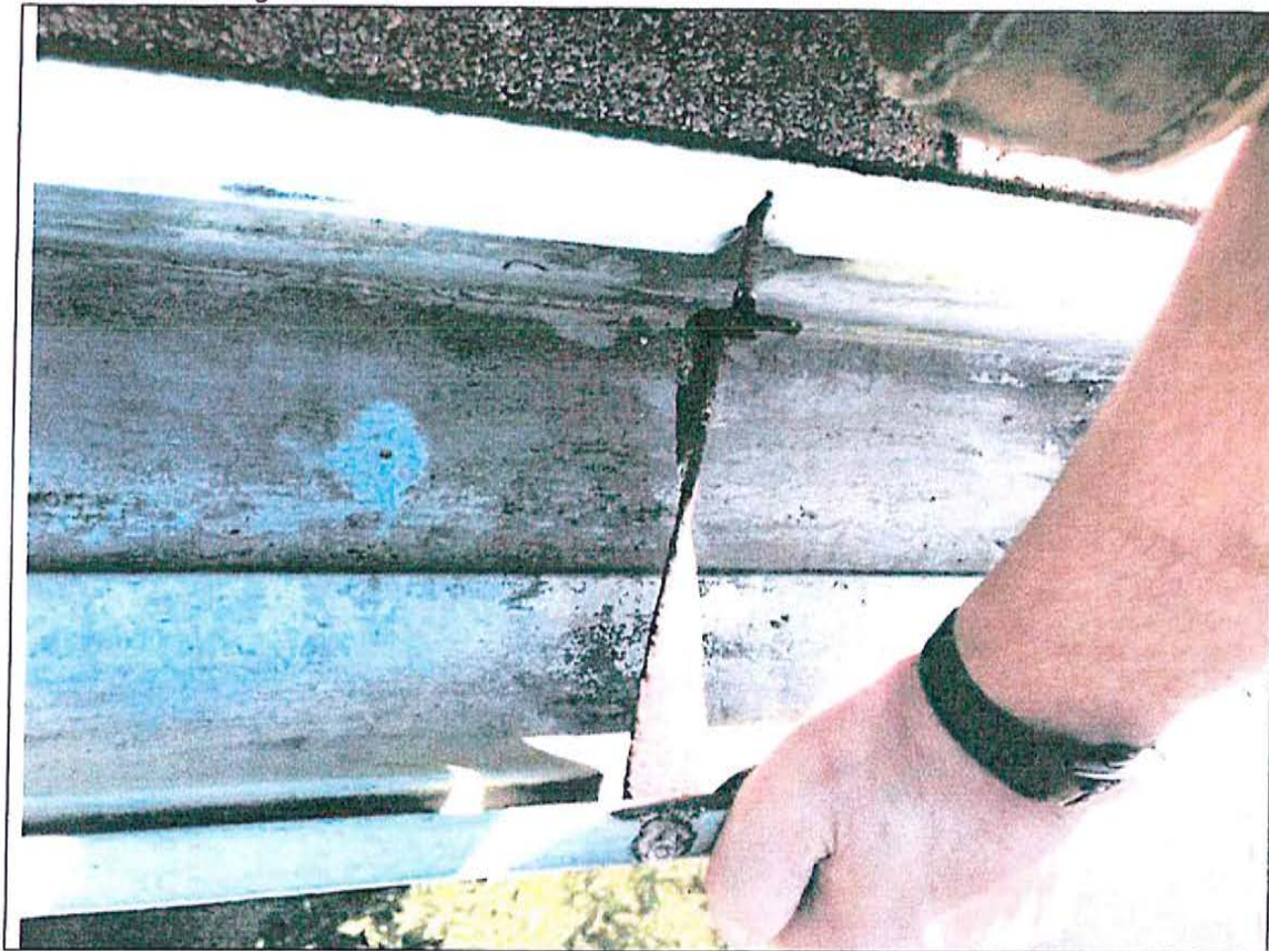
Hanger screw not attached to fascia.
