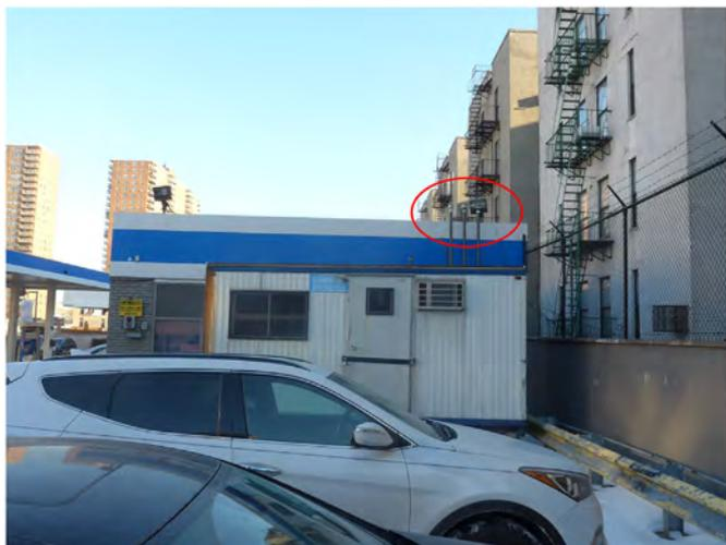
**Fig. 1.** The three vent pipes (enclosed by the red ellipse) on the right side of the convenience store of a gas station are <10 m away from the residential building. (For interpretation of the references to color in this figure legend, the reader is referred to the web version of this article.)
