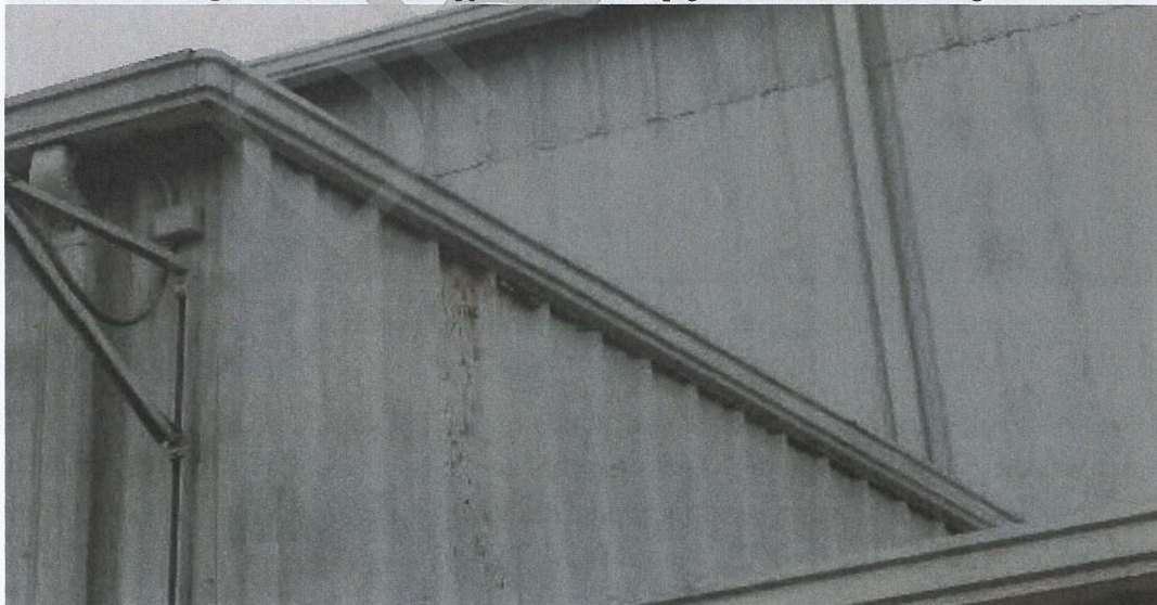
Figure 3: The brown/white-wash coming down below the gutter, classic sign of European starling nest.
