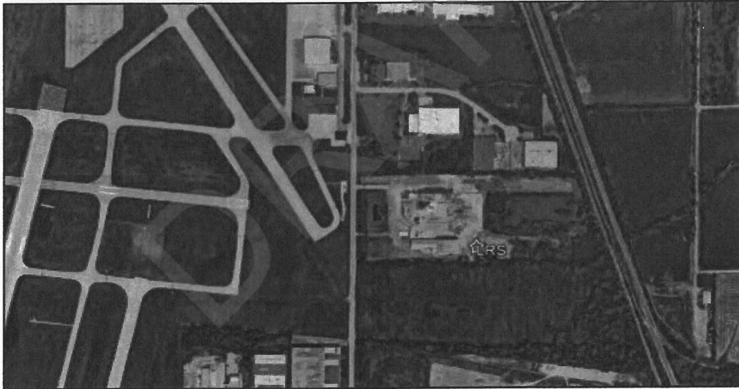
Figure 1: The star is the location of the future MSW transfer station building, inside the LRS boundary.
