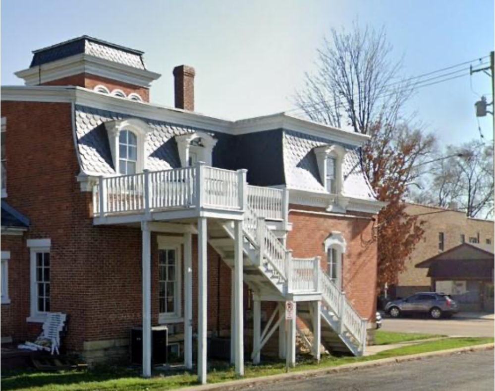
Photographs of the existing site conditions
